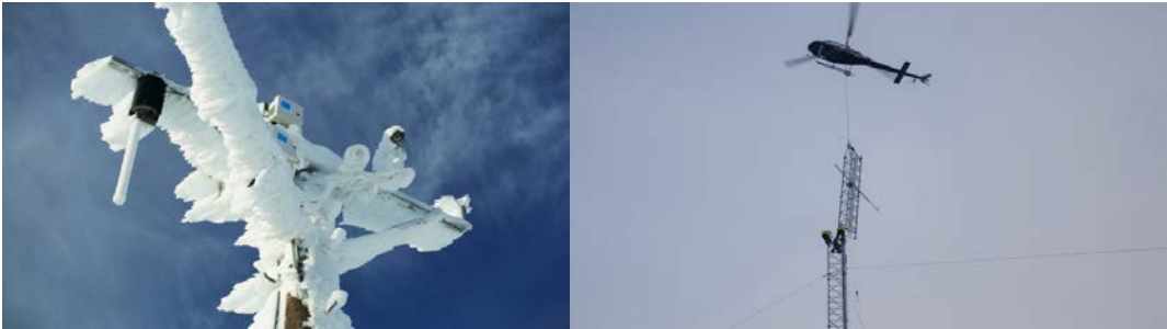
Figure 3 : A) Icing forecasts equipment B) Installation of masts © Kjeller Vindteknikk
